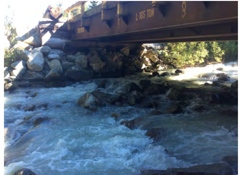
Right Bank Abutment when facing downstream
