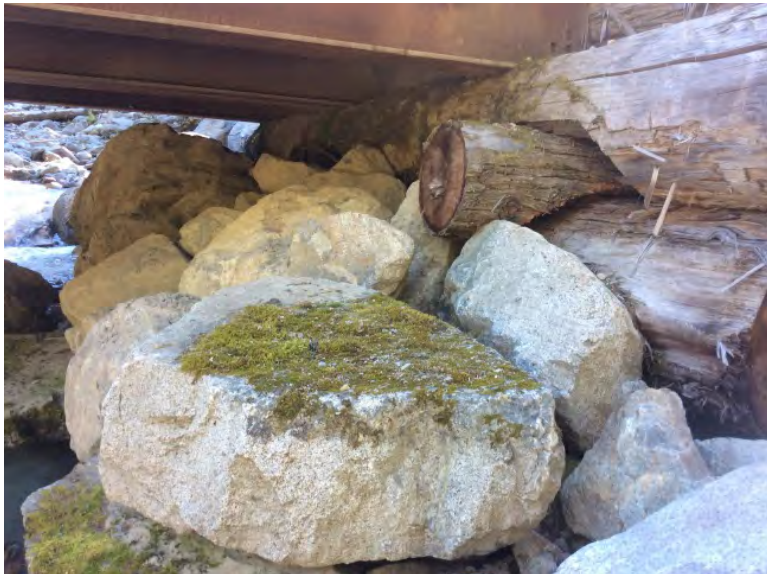
Left Bank Abutment when facing downstream
