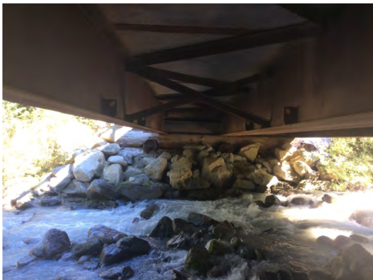
Right Bank Abutment when facing downstream
