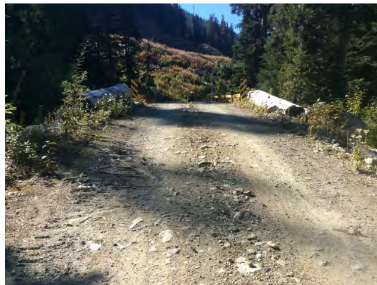
Approach from Right Bank when facing downstream
